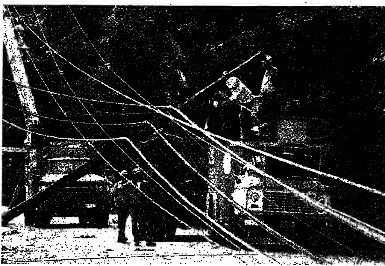
Crews from the Long Island Lighting Company and the New York Telephone Company working on one of seven poles that went down on Shore Road, Oyster Bay, L.I., when Hurricane Belle struck.
